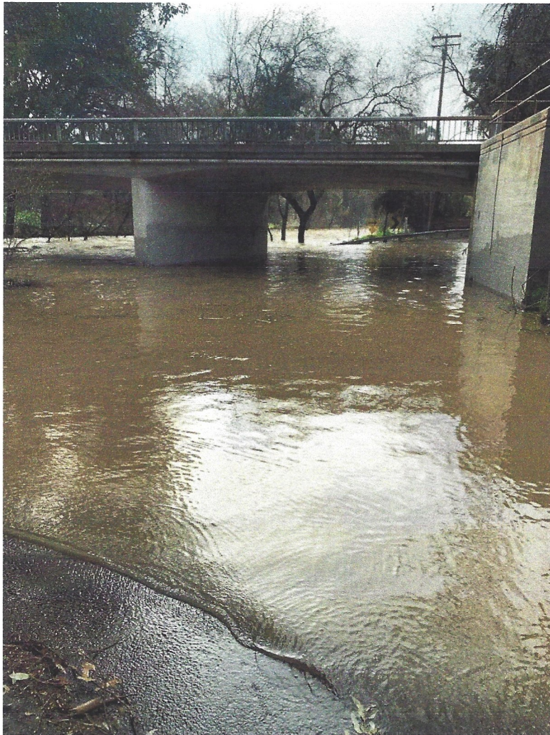
Dry Creek La Loma Bridge at Morton under-pass
