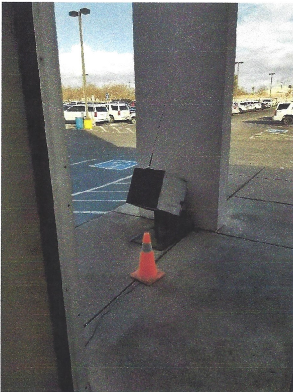
NCS temporary antenna drop.
